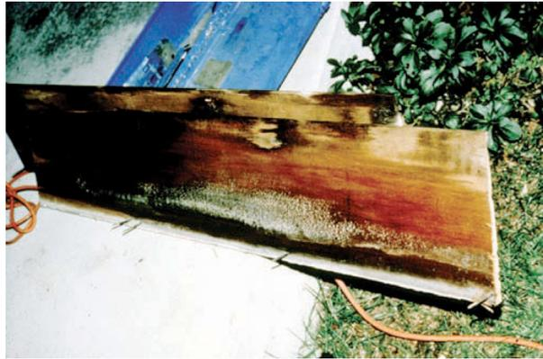
**Photograph 3: Wet Cladding**—Problems with mold and decay were worse on north and east elevations. Problems with peeling paint were worse on west and south elevations. Solar radiation cycled the cladding moisture content more on the west and south elevations stressing the paint. UV cross-linked the paint making it less flexible. Less flexibility, more movement on the south and the west led to the peeling paint. Less energy on the north and the east led to the mold and the decay.
