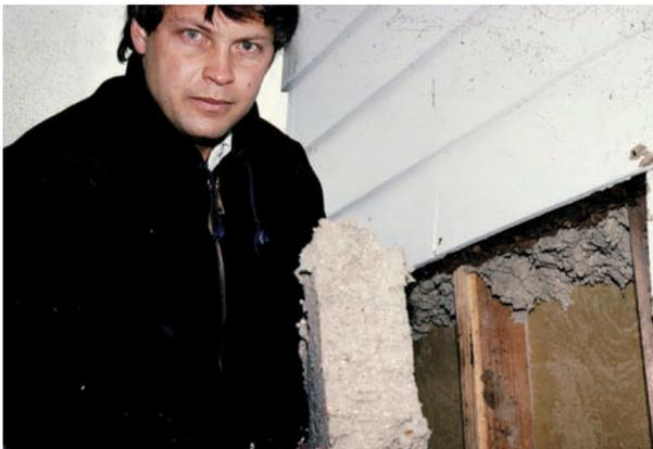
**Photograph 2: Retrofit Cellulose Cavity Insulation**—Dry blown cellulose packed into exterior wood frame walls. Injected from the exterior at top of cavity. This author, very young at the time, amazed at how well the insulation worked. Cavities were dry when opened.
